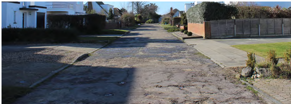
Figure 102 Uneven road surfacing
