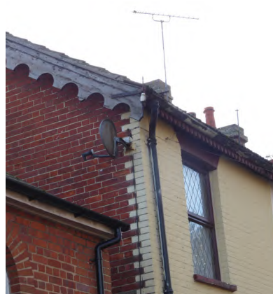
Figure 73 Decorative eaves and corner brick detail
