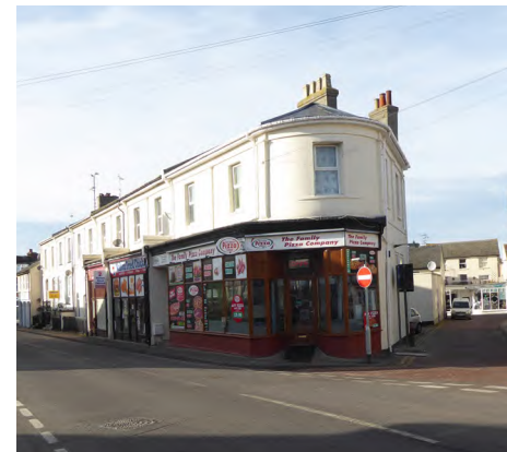
Figure 79 Example of commercial building on corner plot
