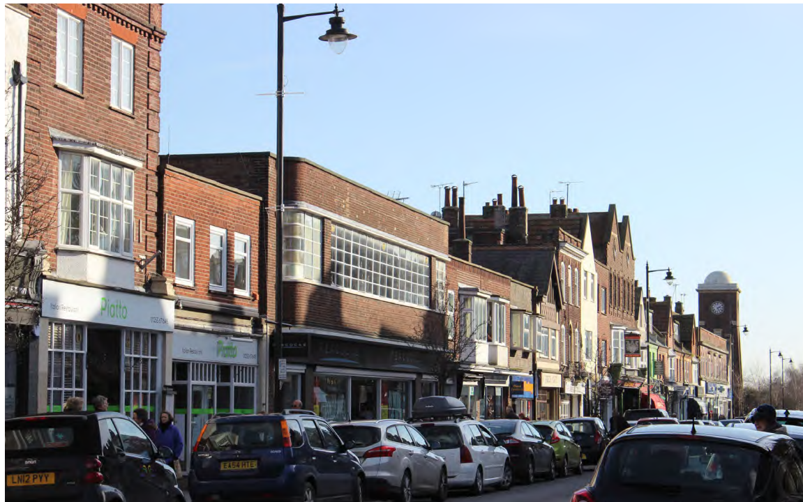
Figure 37 Brick frontages on the east side of Connaught Avenue, with varied rooflines and gables fronts to the south
