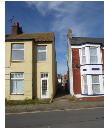
Figure 74 Small spaces between buildings
