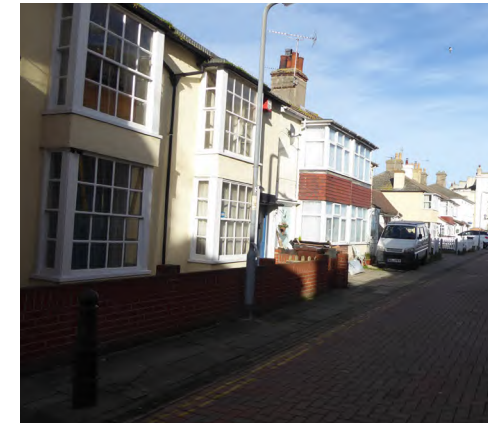
Figure 84 View along Suffolk Street
