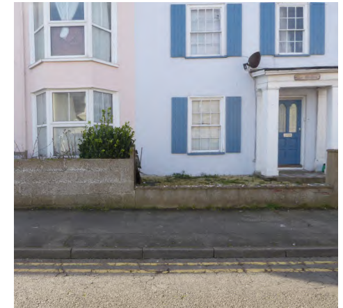
Figure 97 Example of boundary wall replacement
